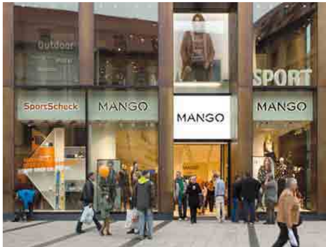
Joseph Pschorr-Haus in bester Lage der Neuhauser Straße: COMFORT konnte neben Forever 21 Mango den bislang weltweit größten Store in dieser High-End-Projektentwicklung vermitteln./Joseph Pschorr-Haus in a prime location on Neuhauser Strasse: In this high end project development, COMFORT was able to broker to both Mango and Forever 21 their largest stores worldwide.
